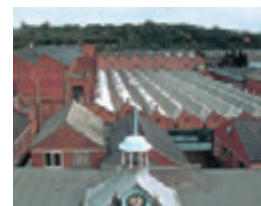
NSK Newark Plant
