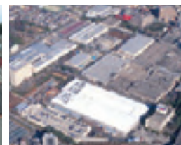
NSK Fujisawa Plant
