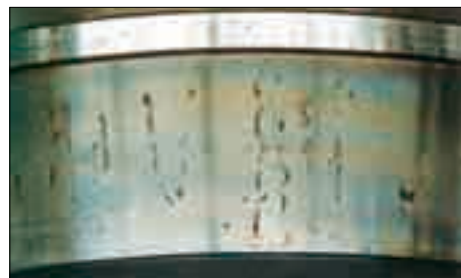
Rust and corrosion
