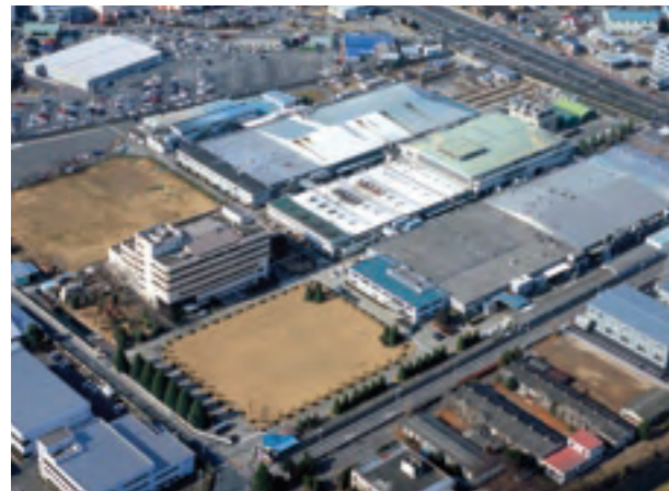
NSK Precision Co., Ltd. Maebashi Precision Machinery and Parts Plant
