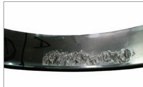
Photo 1-10 Part: Enlargement of raceway surface in Photo 1-9 Symptom: Flaking of one side of the raceway Cause: Excessive pressure due to misalignment
